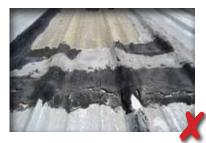
This type of seam repair is found often on metal roofs. Unfortunately asphalt patches become dry and brittle and leaks re-appear quickly.
