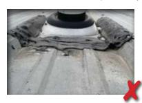
This type of asphalt repair quickly breaks down and pulls away from the roof, breaking the leak proof seal.
