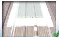
This is a proper repair for a metal roof at overlap seams. The product is flat allowing water to flow freely and remains flexible.
