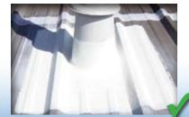
This is a proper repair for metal roof penetrations. The products are very flexible and remain flexible even after curing.
